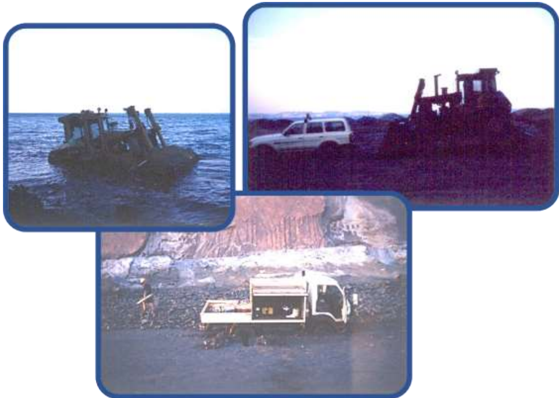
The bogged truck leads to a bogged dozer about to go under for the second time. The dozer was back on dry land prior to having the exhaust refitted.
